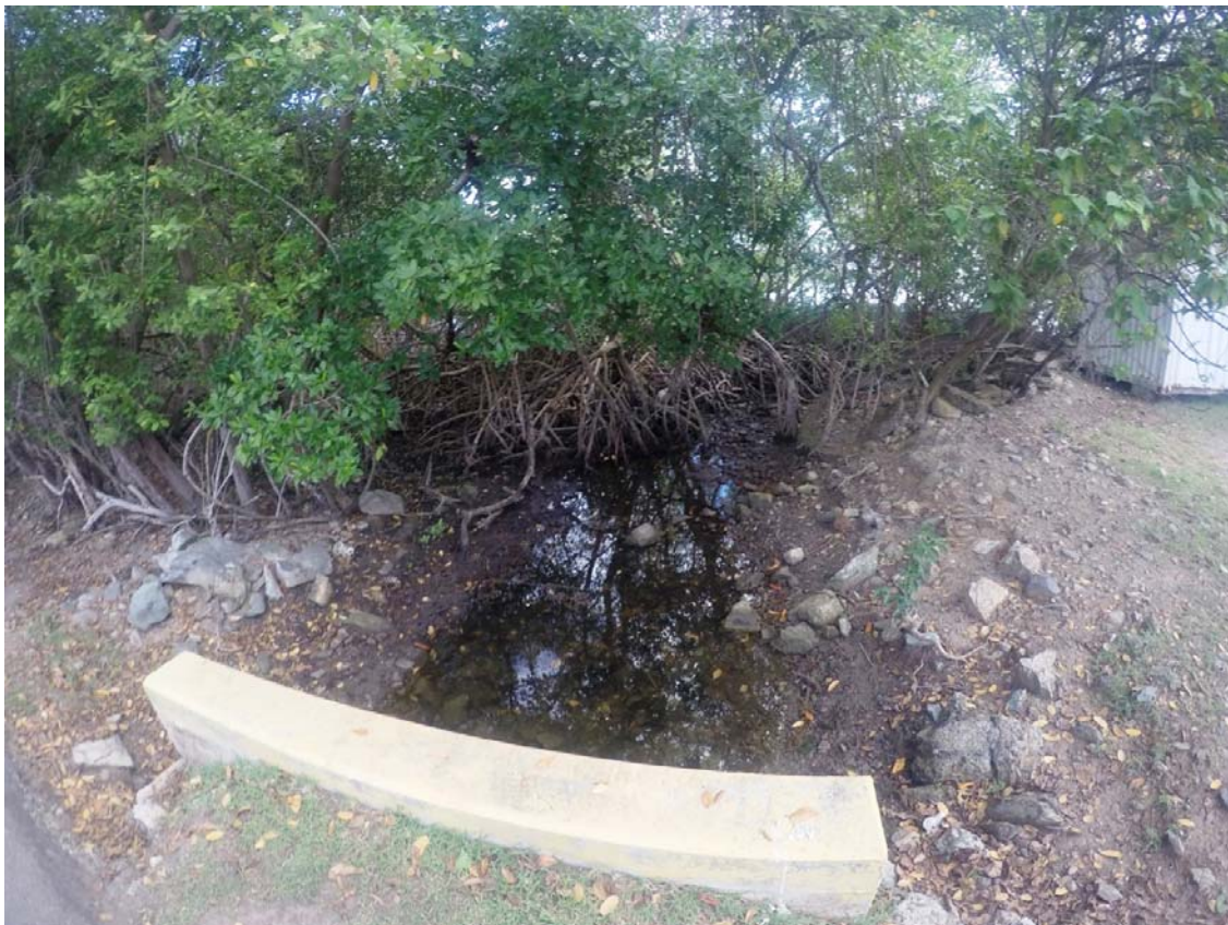
Culvert at base of ghut with freshwater discharge from Coral Bay watershed that discharges directly into red mangrove wetland in the northeastern corner of Coral Bay.
