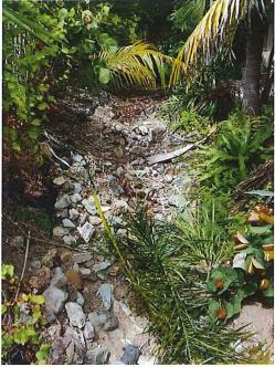
At the intersection of Route 107 and Harold's Way there are several areas of concern that need maintenance. The culvert under the road needs cleaning at both ends as they are partially clogged with debris and vegetation as shown below.
